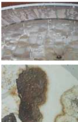
Floating tank top - application over existing corrosion post high pressure water washing & hand preparation
