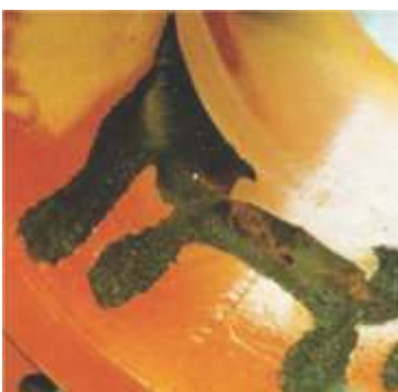
Severe Cavitation Damage
