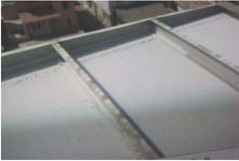
Metal roof protection & sealing
