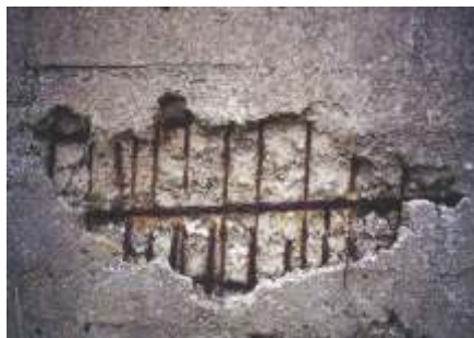
Protective coating for "deteriorated", damp concrete
