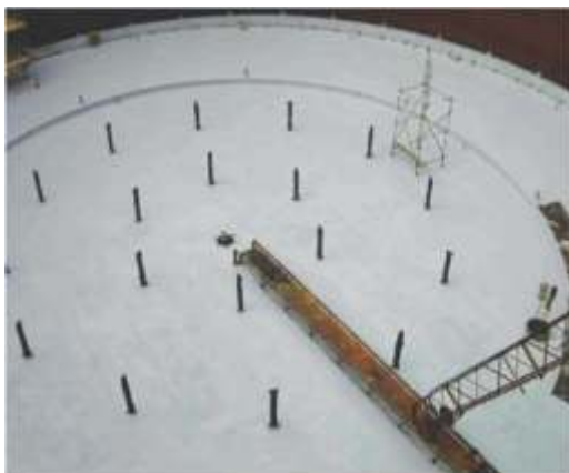
Floating tank top - application over existing corrosion post high pressure water washing & hand preparation
